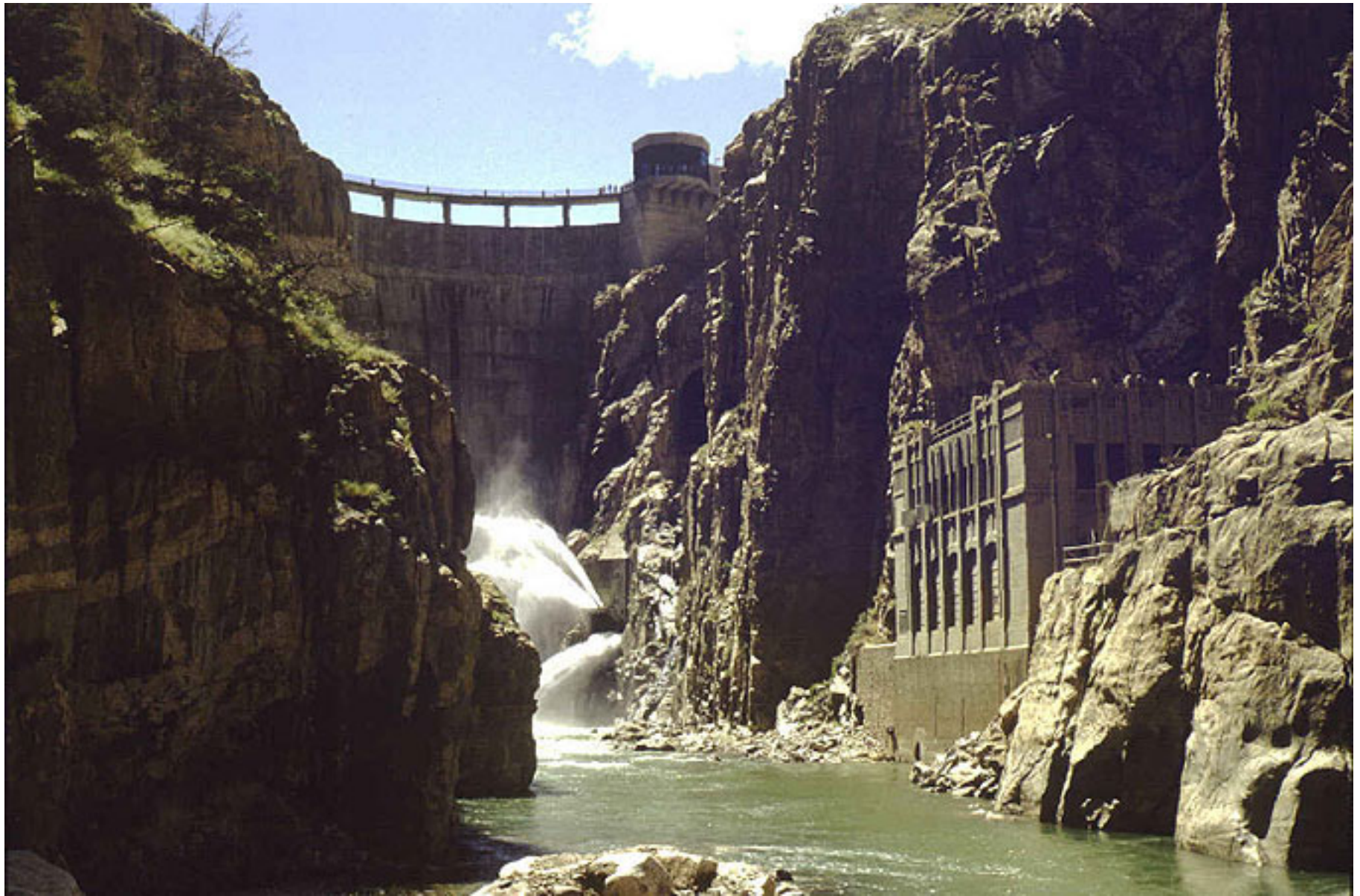
Archean gneiss and granite abutments of Buffalo Bill Dam. Image from: https://upload.wikimedia.org/wikipedia/commons/7/7b/BuffaloBillDam.jpg ( https://upload.wikimedia.org/wikipedia/commons/7/7b/BuffaloBillDam.jpg )
